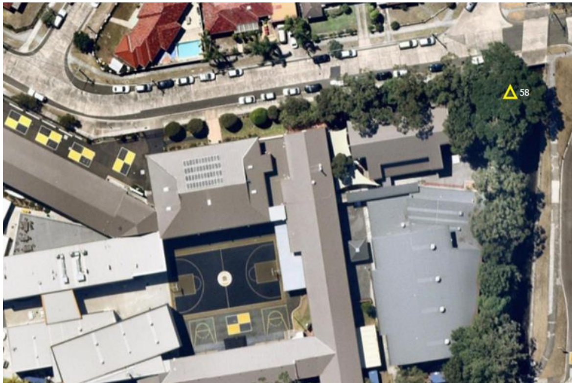
Figure 5. Aerial image showing location of High Retention Value Trees. Note that icon colour indicates trees current risk rating (not Retention Value). Tree attributes are to be obtained from Appendix C – Tree Assessment Data. (ArborSite, 2019).
